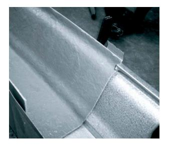
3. In the 3rd photo, the radius gutter slides into the existing gutter up to the point where the flap was cut. 800 Fulgham Ste. #24 Plano, TX 75093 214-215-8369
