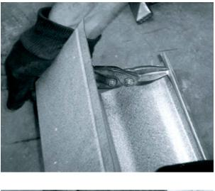
1. First, prepare the existing gutter. From the end, measure in 1  $1/2^{"}$ . At this mark use your metal snips and cut the front lip of the gutter (where the hidden hanger fits into), including the top.
