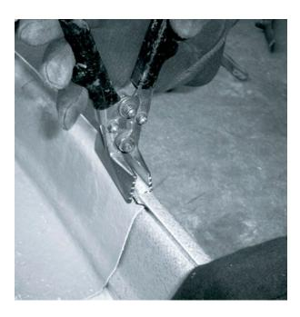
4. With the bending pliers, fold the cut flap over the radius gutter and crimp down to hold tight.
