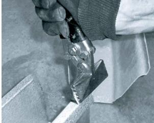
2. With a pair of bending pliers, bend up the inch and a half flap, so the radius gutter can slide into the existing gutter.
