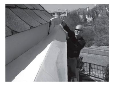
3. Take a Sharpie or magic marker and duct tape it to the end of a 4 to 6 ft. stick.
