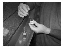
2. Use one bottle of resin and 2 ml of hardener for each lap joint. Remove the lid from the resin bottle and set to the side. Squeeze 30 to 35 drops of hardener using squeeze bottle. Replace Resin cap and shake for about 10 seconds.
