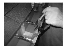
3. Pour about 1/4 of the resin hardener mixture on to the lap joint and spread with brush along front and back. Apply a strip of fiberglass on to the lap joint, making sure half is on the lap joint and half is on the adjoining piece. Pour the remaining amount of resin on to the lap joint and spread evenly with the brush, making sure to dab the top, the front, and the back bead. Spread the excess resin along the inside of the gutter.
