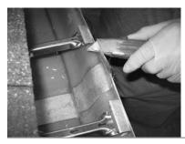
4. Let lap joint fully cure before removing clamp. (When it is no longer tacky to touch) Once the piece is bound, fill the outside seam with the Easy Sand Polyester Finishing Putty supplied with your order. It dries in about 3 minutes, and ready to sand in 10 minutes. Use a 220 grit sand paper to achieve a smooth transition.
